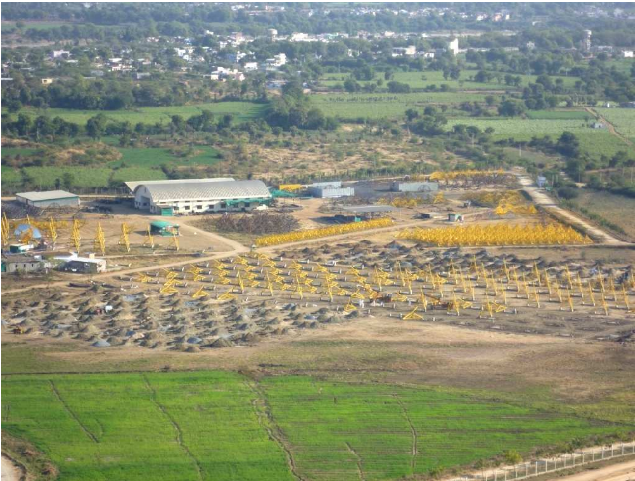
Solar field with fabrication facility and part foundation/installation (Jan.2012)
